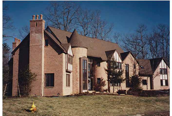
[GAF Ultra Timberline Architectural Shingles and copper flashings were used for Slingerlands, NY home]
