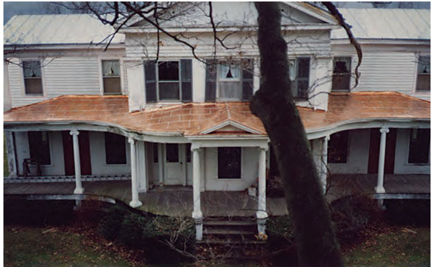
[Ornate Copper Entrance Porch Roof With Built-in Gutters On An Old Middleburg Colonial]
