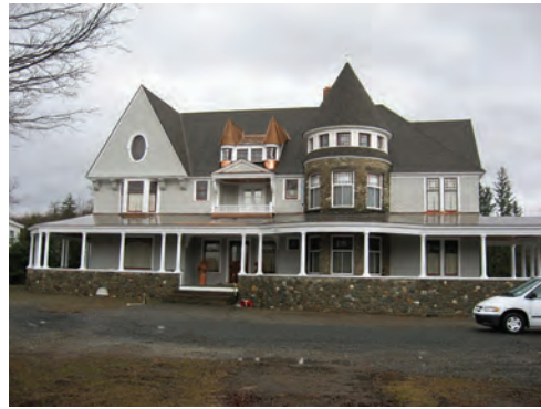
[Flat locked & soldered copper was selected for the low pitched roofs on this 1894 Queen Anne Victorian, while center small turrets were formed into standing seam.]
