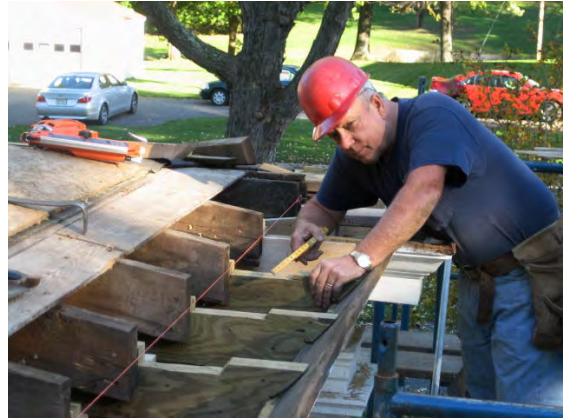
[Staats checks alignment and pitch for a built-in gutter/terne roof restoration.]
