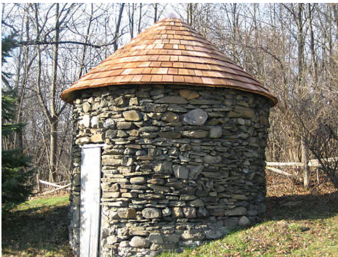
[24" Taper Sawn Cedar Wood Shingles were selected for this 1900 turn of the century stone well house]
